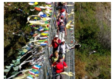
Crossing Hillary Bridge
